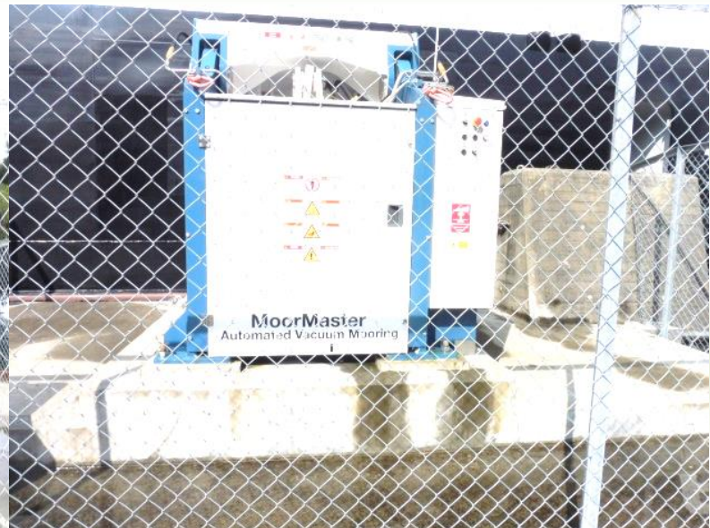
Vacuum operated suction cups has replaced mooring ropes.
