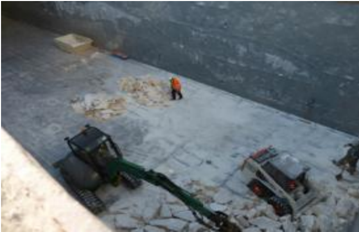
Back-hoe with a hammer attachment at work.
