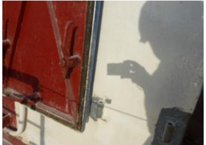
Sealing rubber found in good condition.
