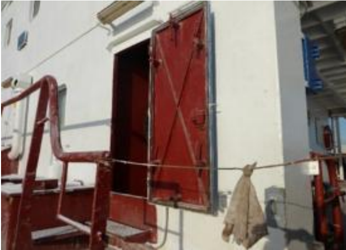
Port side cargo hold entrance.
